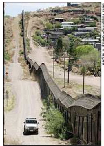
A U.S. border patrol agent drives along the steel wall that separates the U.S. and Mexico.
